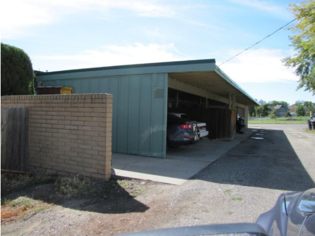
View of covered parking access from alley north of apartment building
