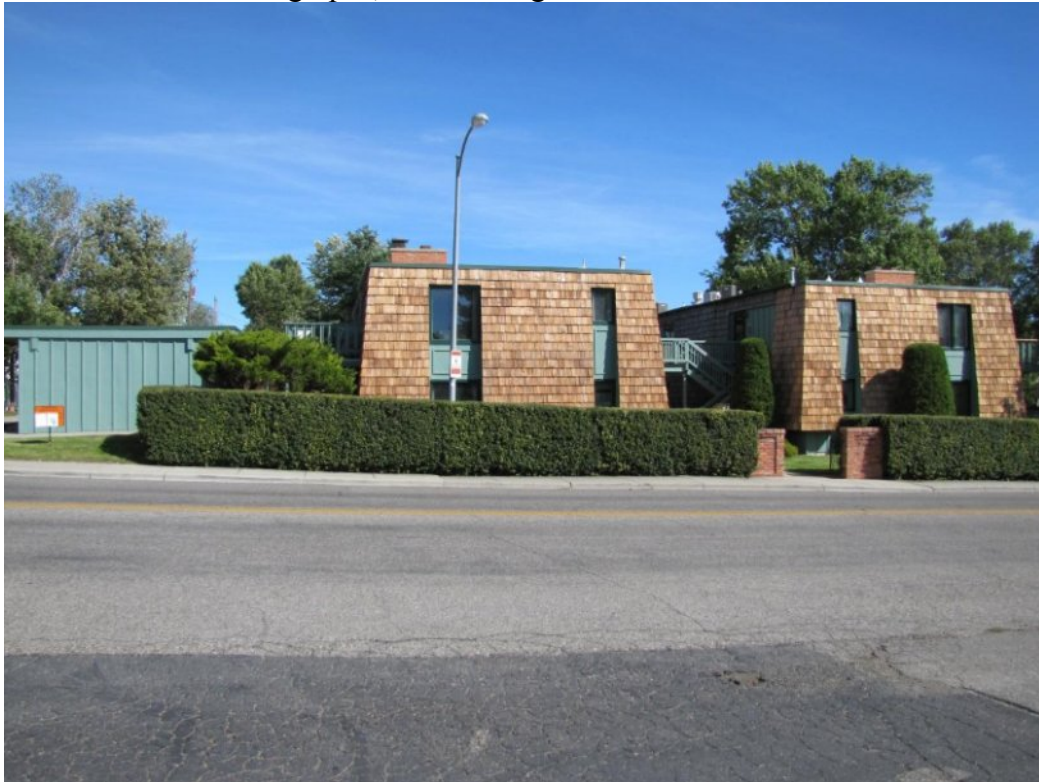
View to the east across 13 th Street West – Subject Property
