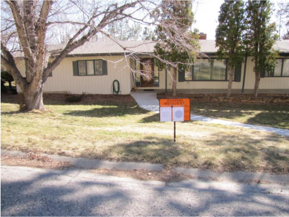
Subject Property from Fairview Place
