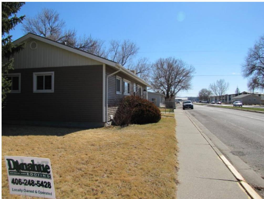
Looking south along face of subject property
