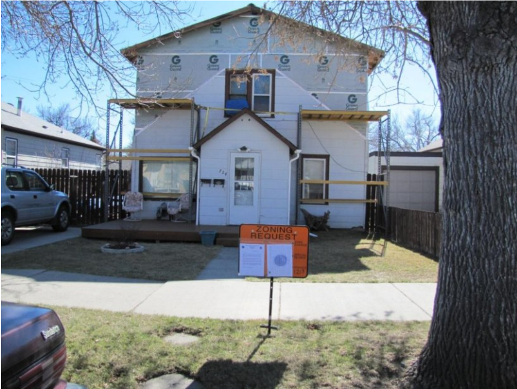
Subject Property from Custer Avenue
