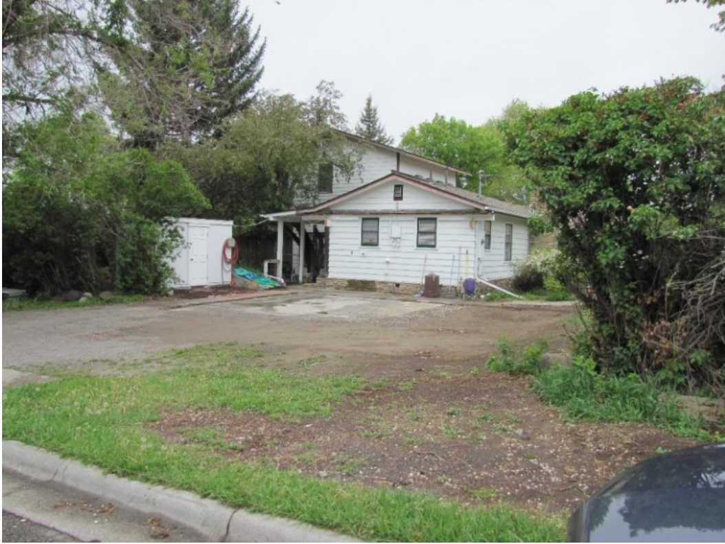
View of east side of dwelling from Dahlia Lane
