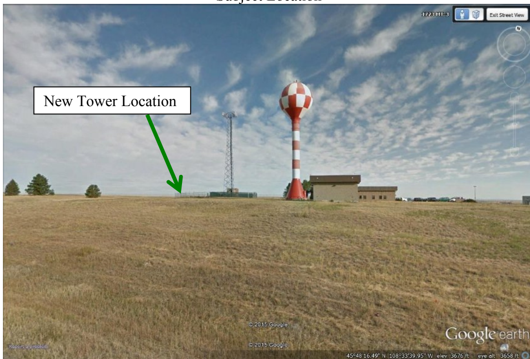
View north from Highway 3
