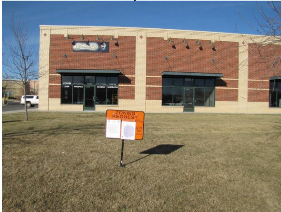
Subject Property from Grant Road
