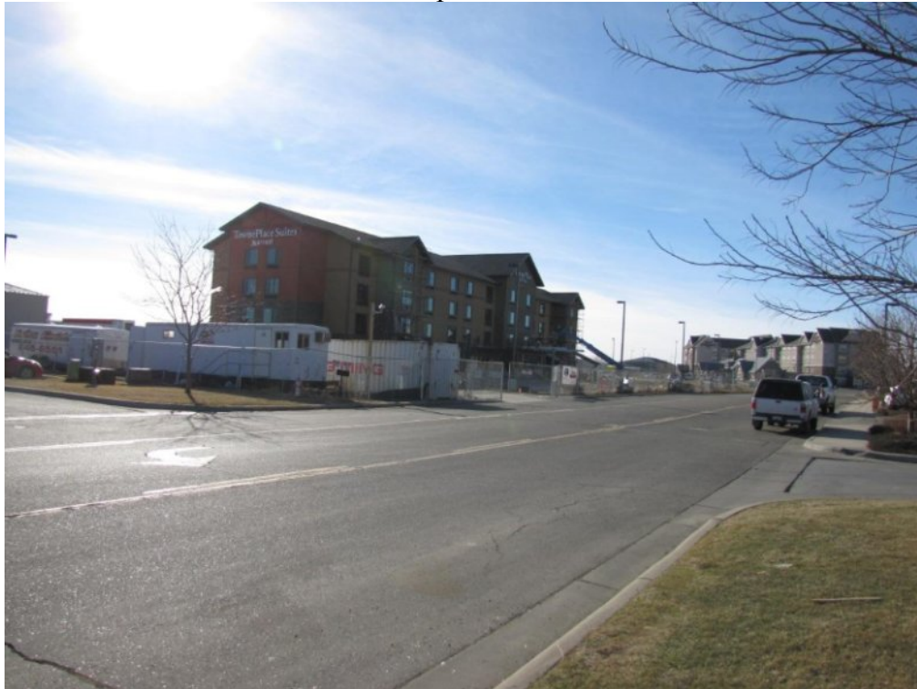
View south and west across Grant Road
