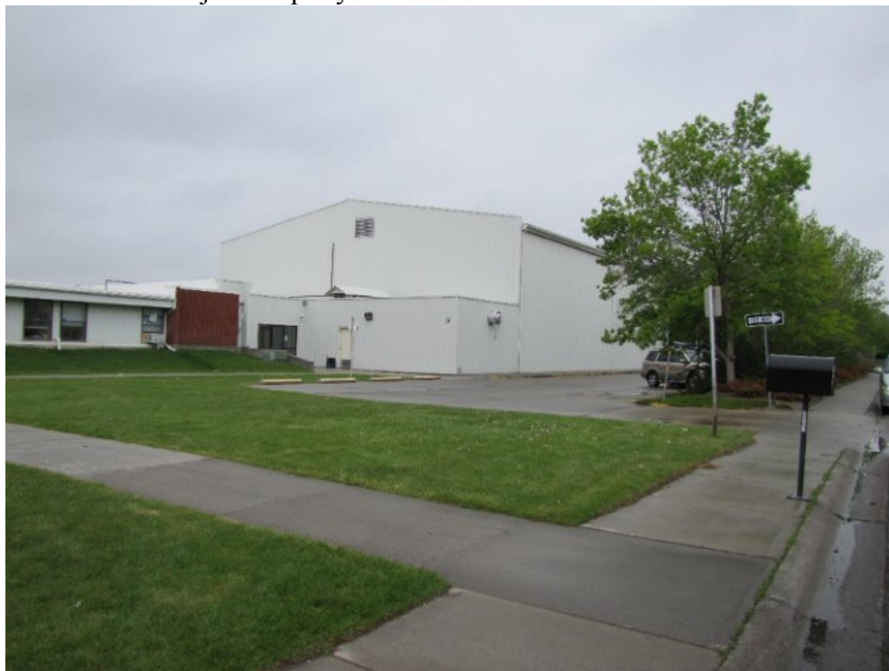
View south and west from Main entrance on Belvedere Drive
