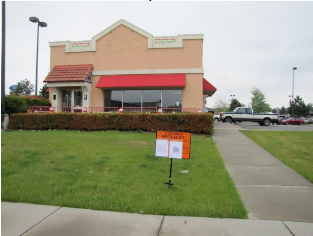
Subject Property from King Park Drive
