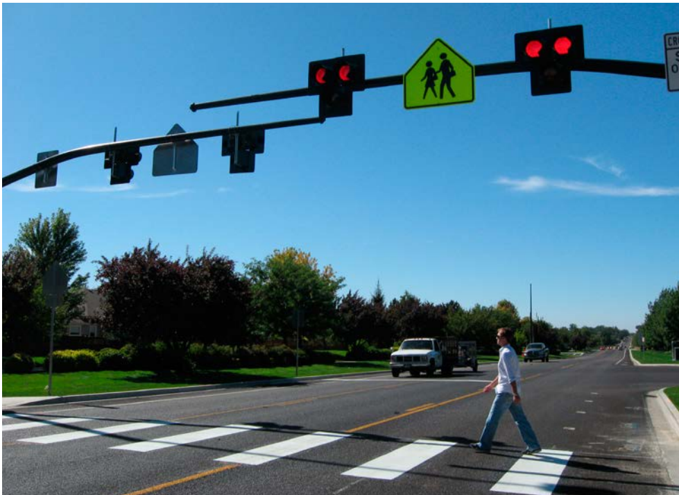
FIGURE 2-21 EXAMPLE OF A HAWK (HIGH-INTENSITY ACTIVATED CROSSWALK). PHOTO FROM ACHDIDAHO.ORG
