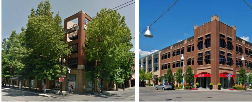
FIGURE 2-35 EXAMPLES OF PARKING STRUCTURES
