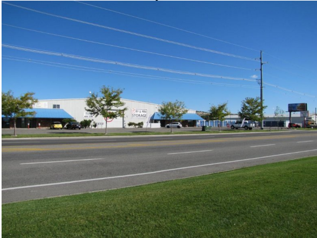
View north west across Grand Avenue from subject property
