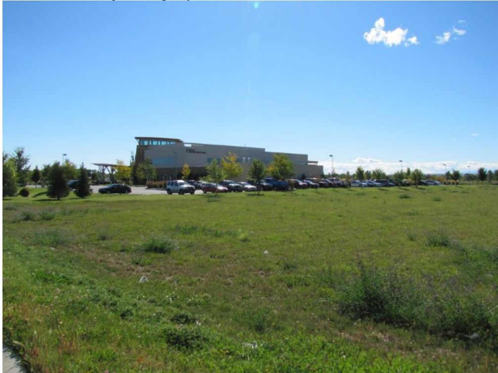
View east of subject property from Grand Avenue
