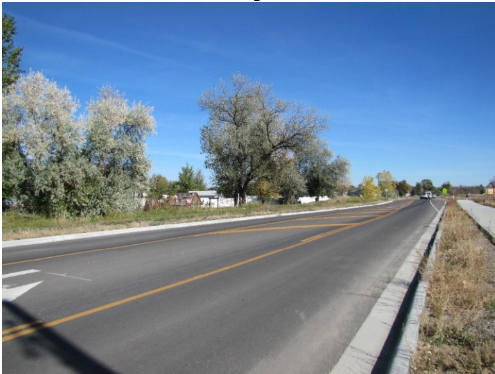
View east along Barrett Road
