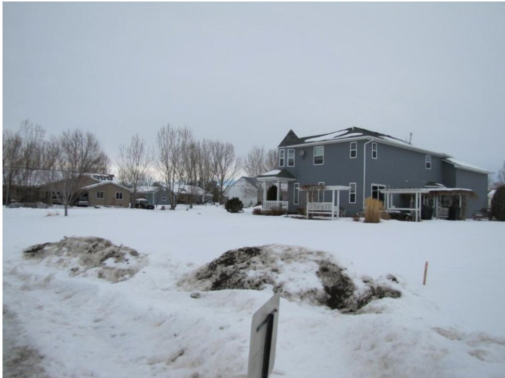
View west of subject property
