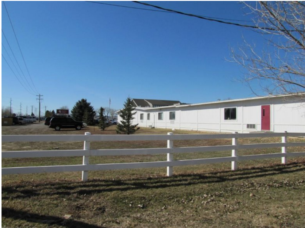
View west at Cornerstone Community Church and School
