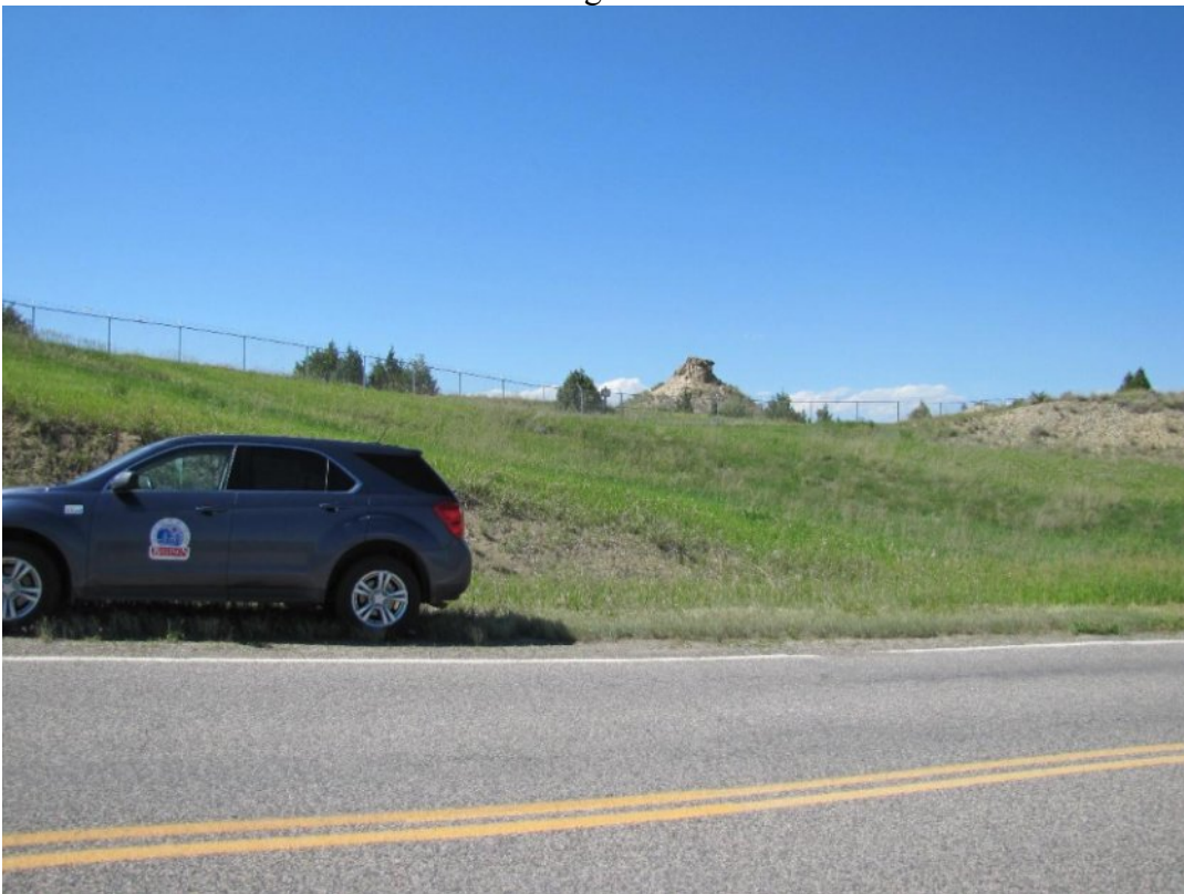
View north across Hillcrest Road
