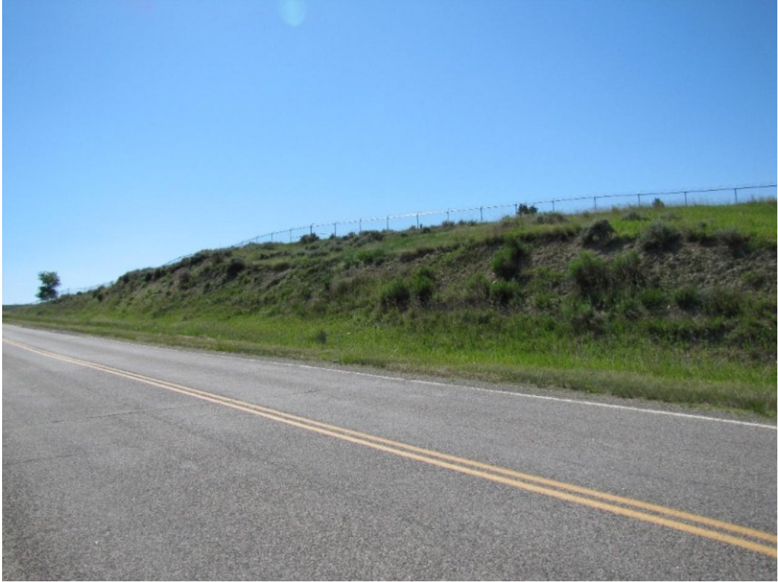
View north west across Hillcrest Road
