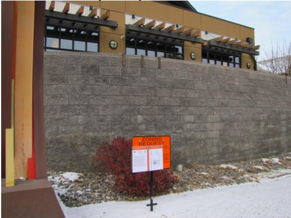
Subject Property – View north from Grand Avenue
