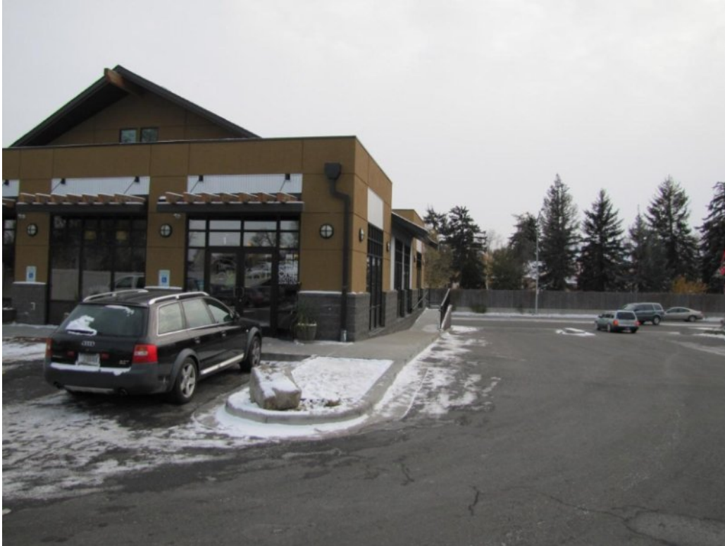
View from existing parking lot south to Grand Avenue
