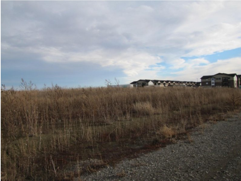
View south and east along 44 th Street West – multi-family apartments under construction
