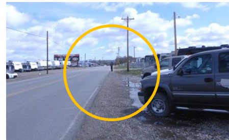
Figure 8: Pedestrians on Old Hardin Road often walk near the travel lane and walk with their back to oncoming traffic, creating a hazard.
