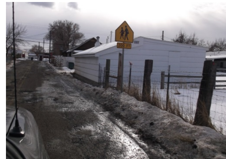
Figure 7: Building restricting the availability of sidewalk placement on the west side of Piccolo Lane
