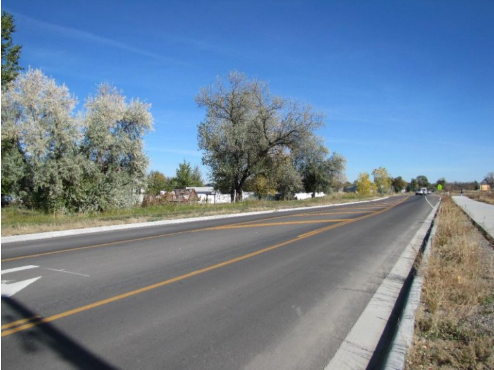
View east along Barrett Road
