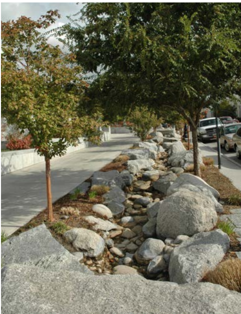
FIGURE 2-3 LANDSCAPED SWALE FOR SURFACE RUNOFF
