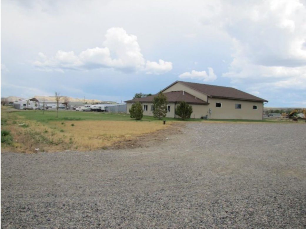
View east of subject property
