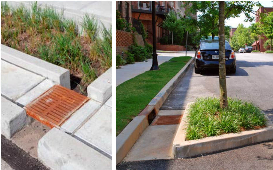
FIGURE 3-2 EXAMPLES OF STORM DRAINAGE IMPROVEMENTS
