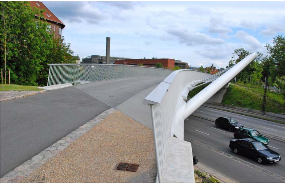
FIGURE 2-20 EXAMPLE OF PEDESTRIAN OVER CROSSING
