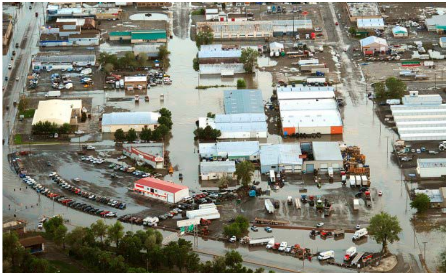
FIGURE 2-6 EXPOSITION GATEWAY AREA AFTER AN EXTREME STORM EVENT- BILLINGS GAZETTE JUNE 20, 2010 (L MAYER)
