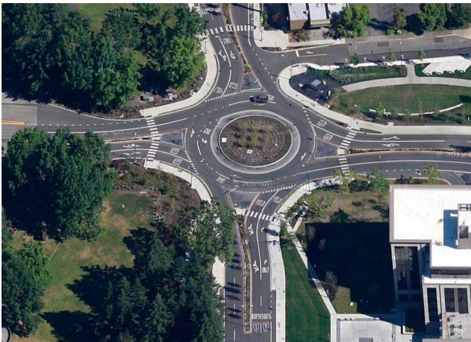
FIGURE 3-6 EXAMPLE OF ROUNDABOUT CONNECTION TO THE INTERSTATE
