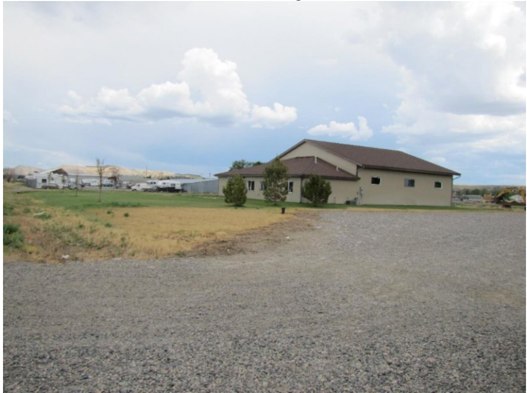
View east of subject property
