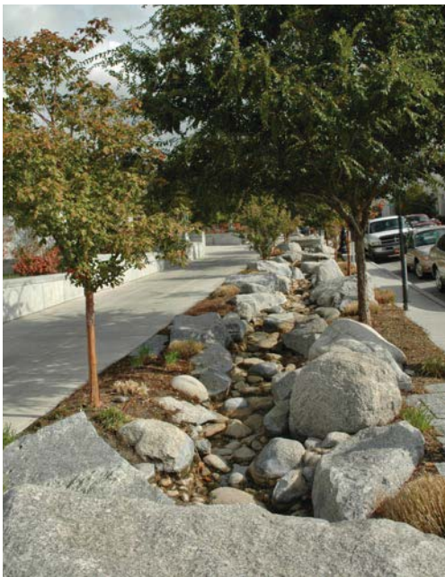
FIGURE 2-3 LANDSCAPED SWALE FOR SURFACE RUNOFF
