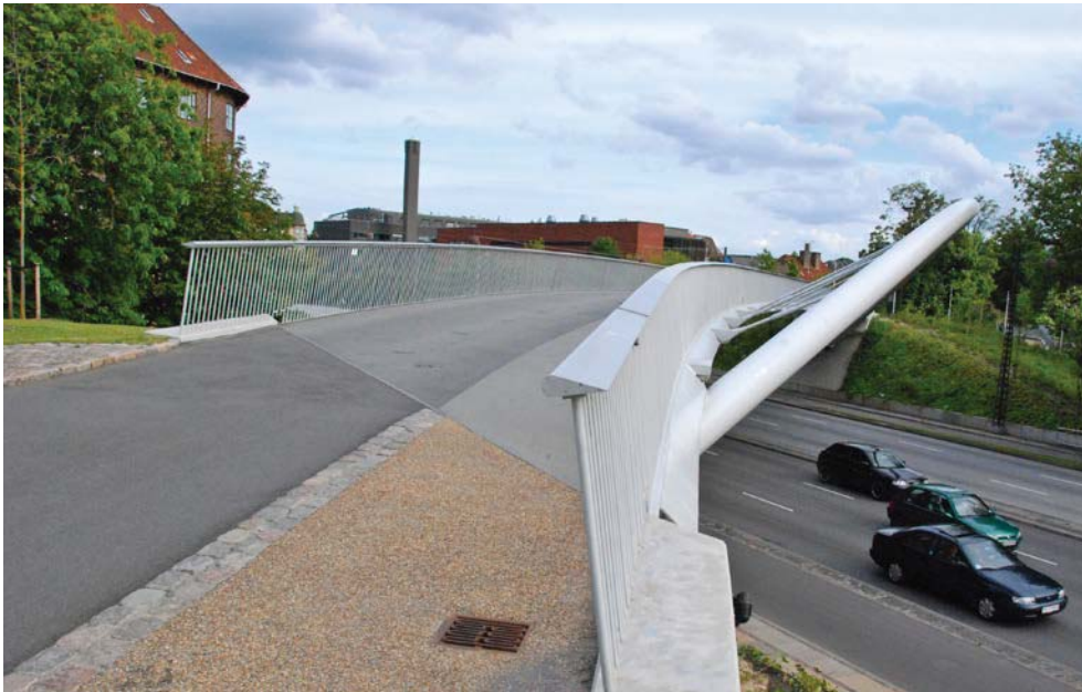
FIGURE 2-20 EXAMPLE OF PEDESTRIAN OVER CROSSING
