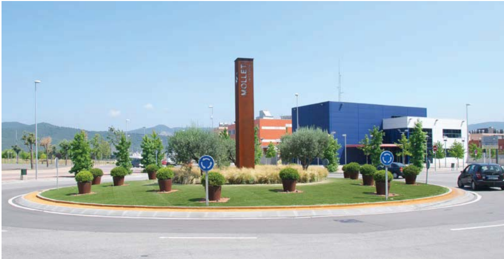
FIGURE 2-27 SPECIAL SIGNAGE WITHIN A ROUNDABOUT
