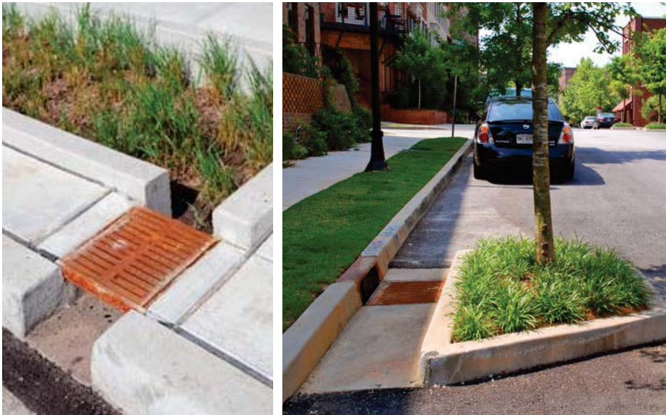
FIGURE 3-2 EXAMPLES OF STORM DRAINAGE IMPROVEMENTS
