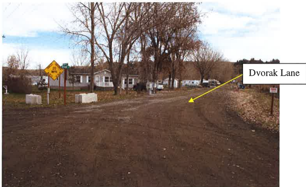
Existing Dvorak Lane Entrance
