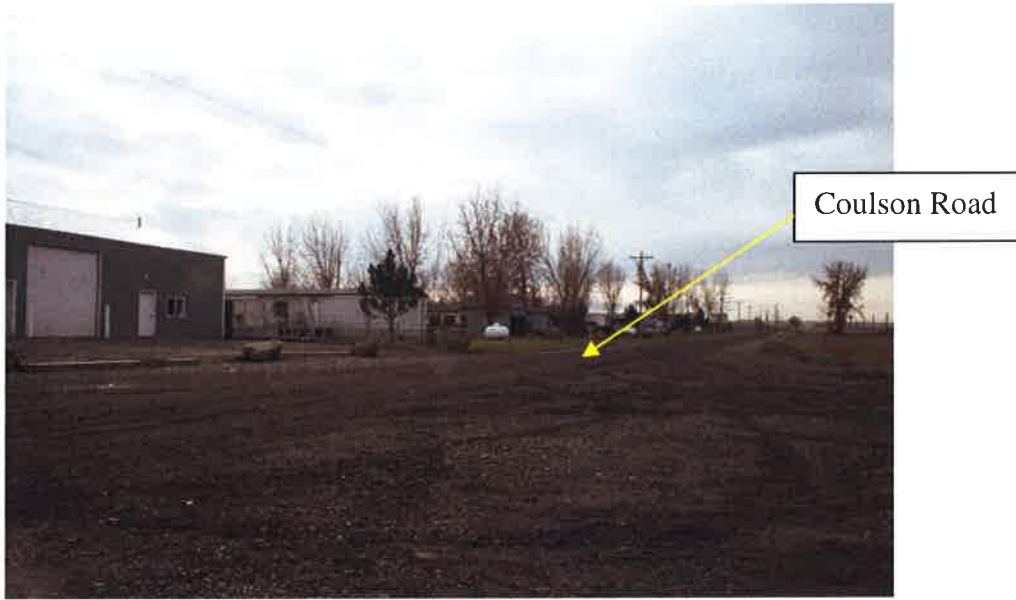
Existing Coulson Road
