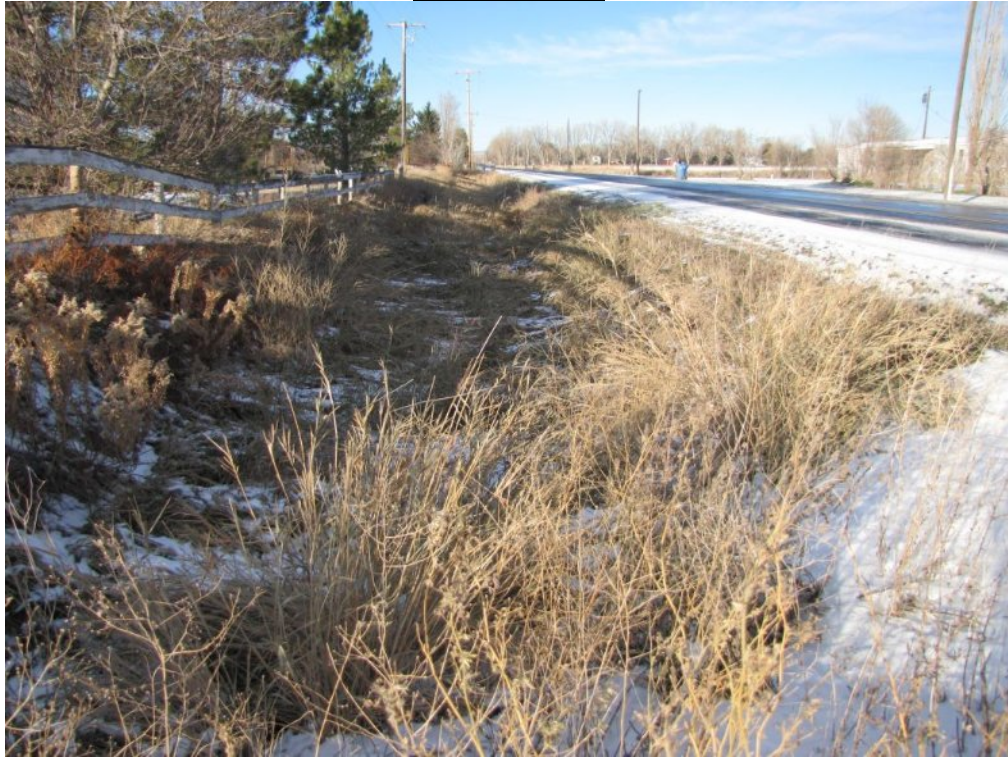
Drainage Ditch from the subject property access looking north
