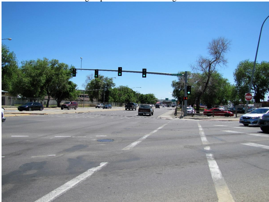
View south along Exposition Drive from signalized intersection
