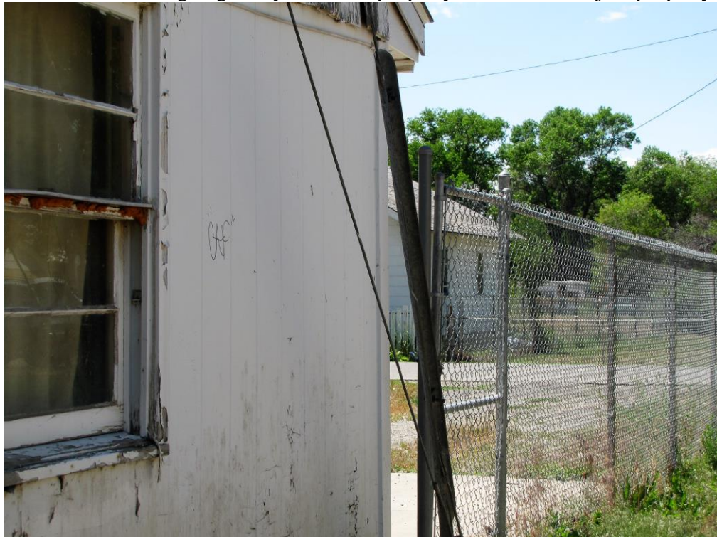
View of house on rear property line west of subject property
