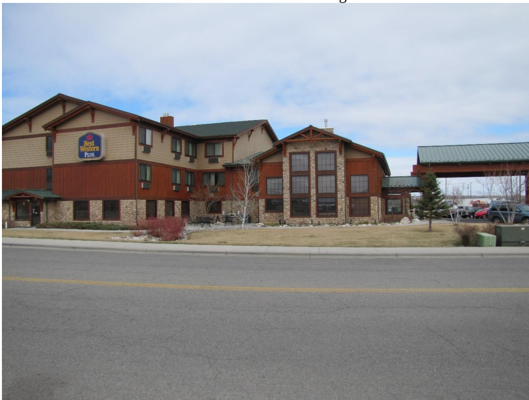
View north across Southgate Drive
