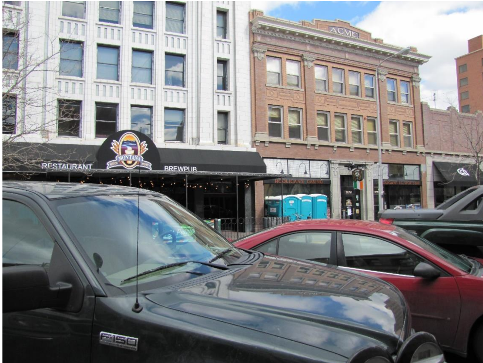
View east across N Broadway
