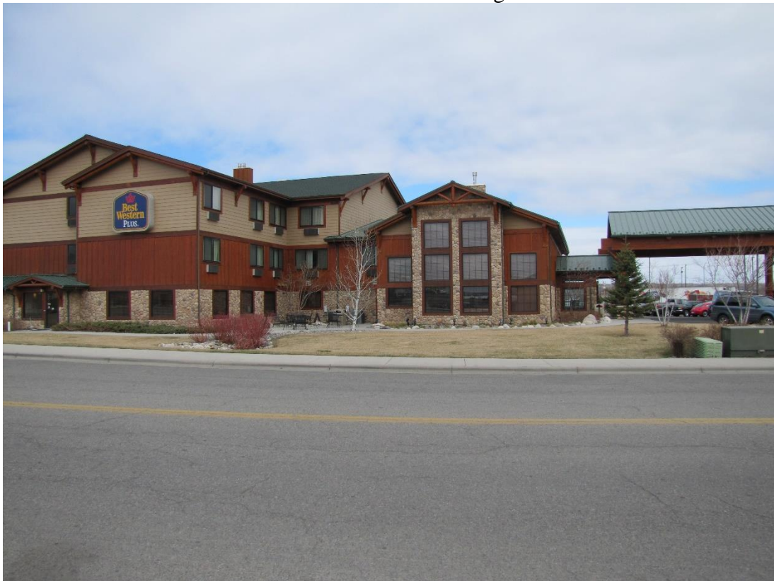
View north across Southgate Drive
