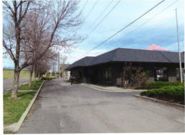
LOOKING NORTH FROM SW
