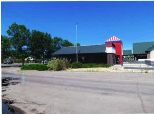
LOOKING FROM SOUTH
