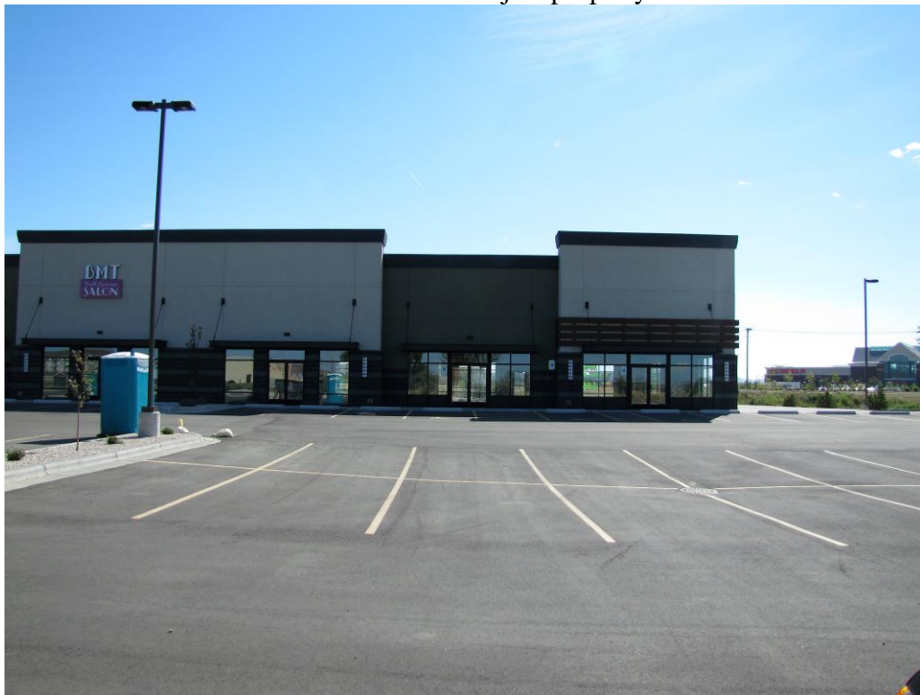
View east across parking lot to subject building on subject property
