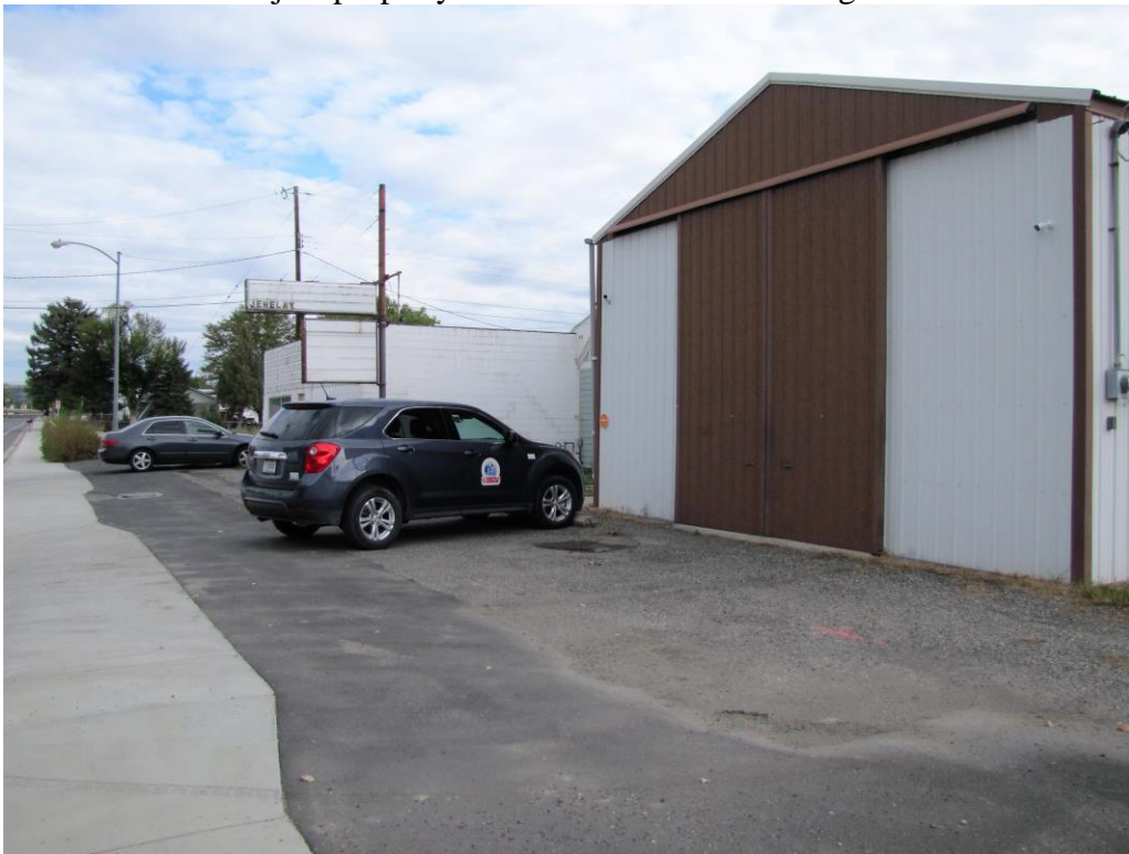
Looking north across existing buildings
