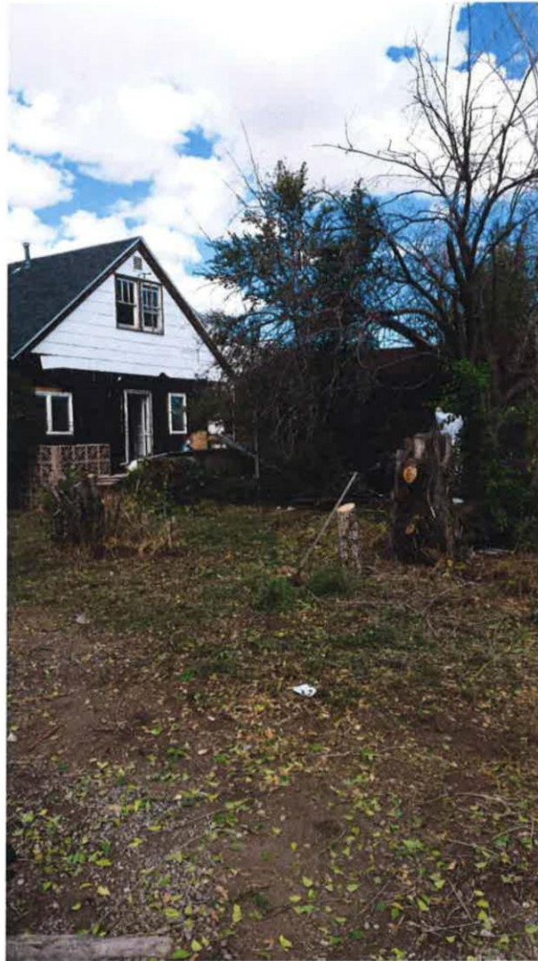
BRUSH REMOVAL FROM LOT 1
