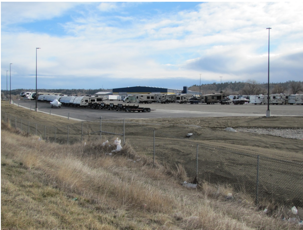
Bretz RV property from the I-90 ROW looking east. Building is in the background and RVs and boars are parked on a portion of the paved storage and sales area.
