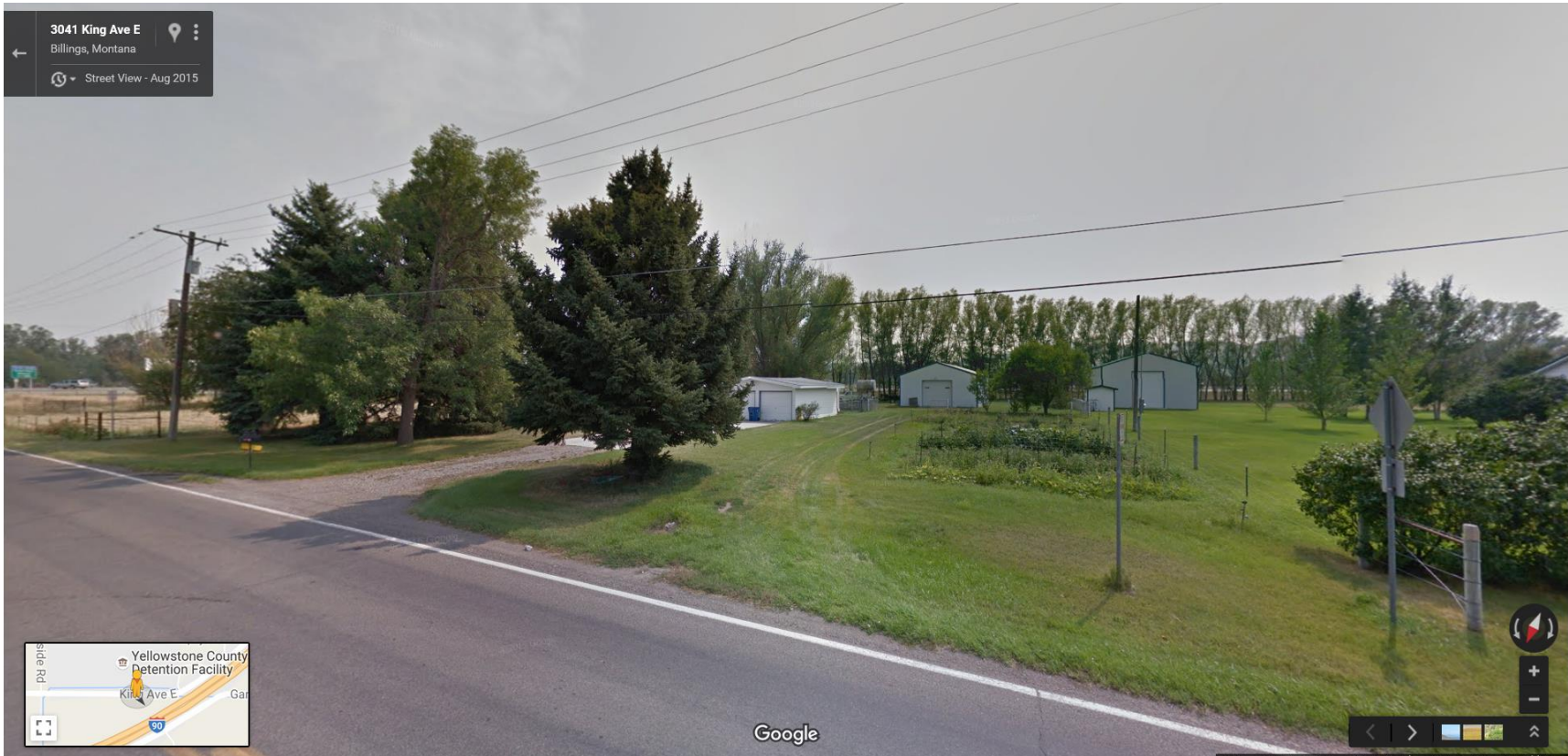
View south east across King Avenue East – 3150 King Ave East
