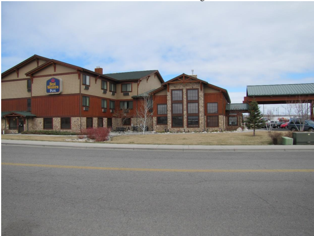
View north across Southgate Drive
