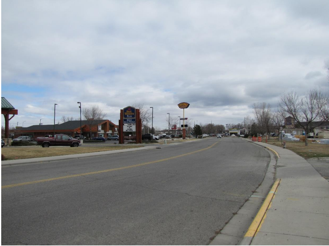
View north and east across Southgate Drive
