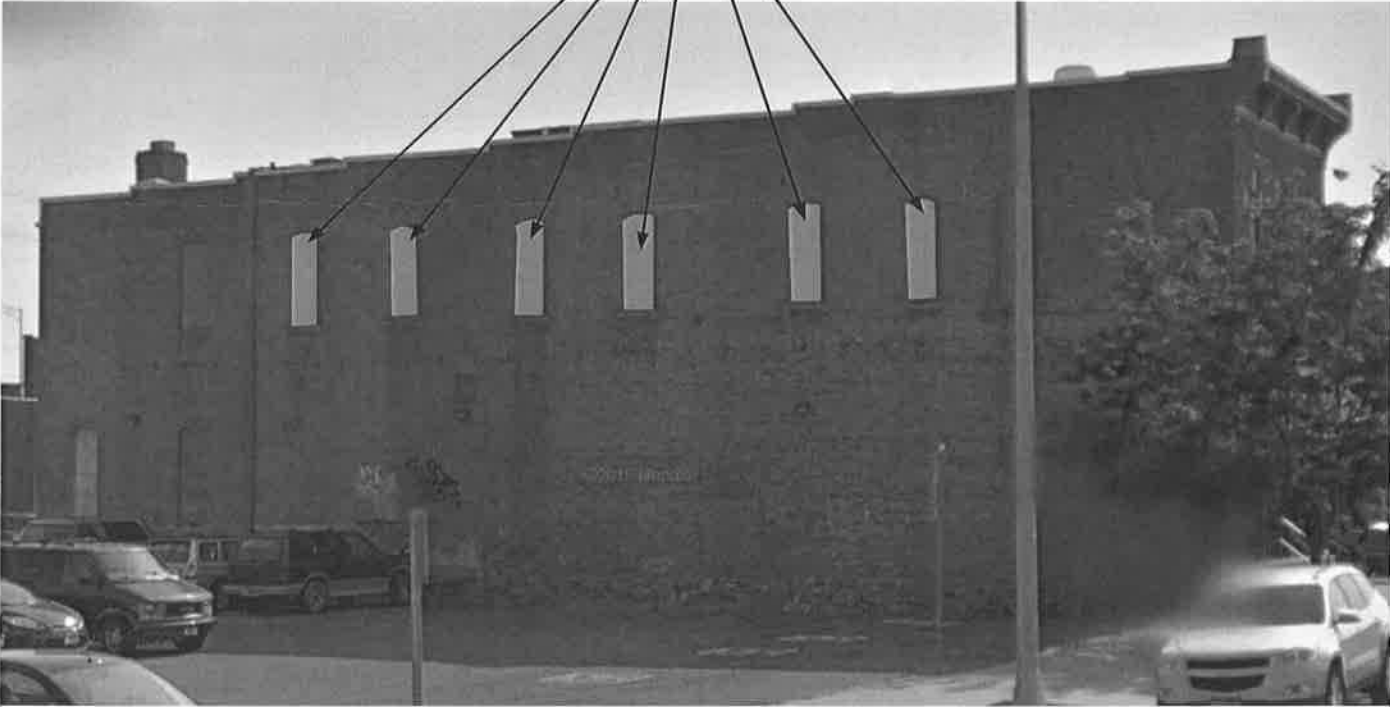
East-side of L&L building
