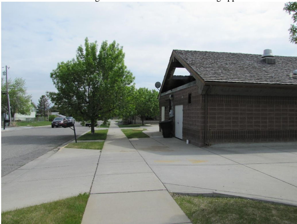
View south along Henesta Drive from intersection with Rosebud Drive
