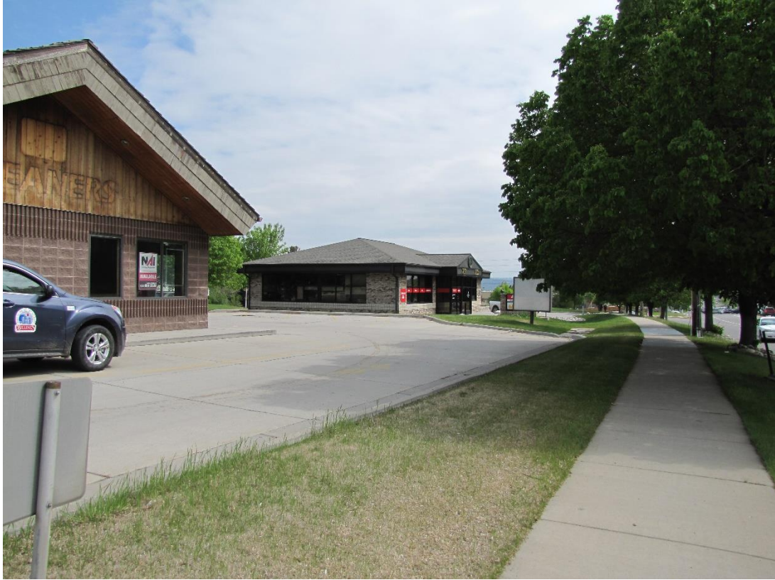
View south along S 24 th St West
