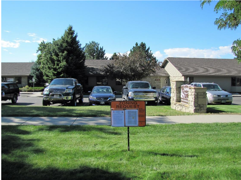
Subject Property from Rimrock Road
