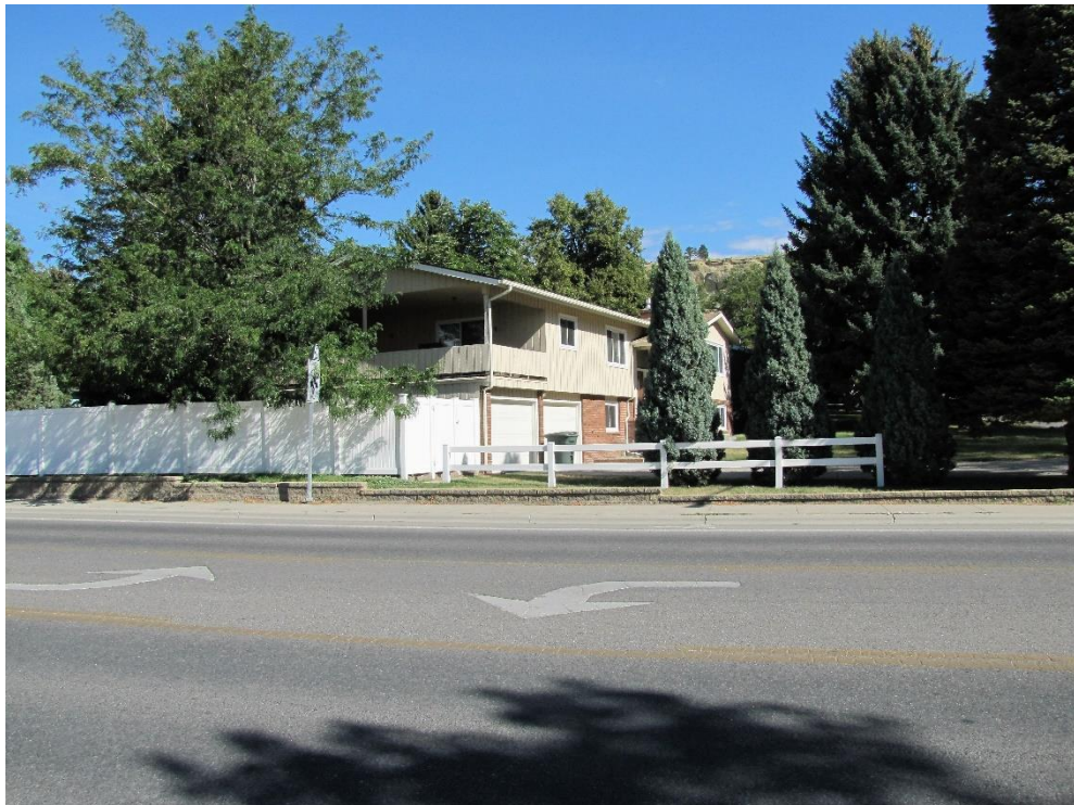
View north across Rimrock Road
