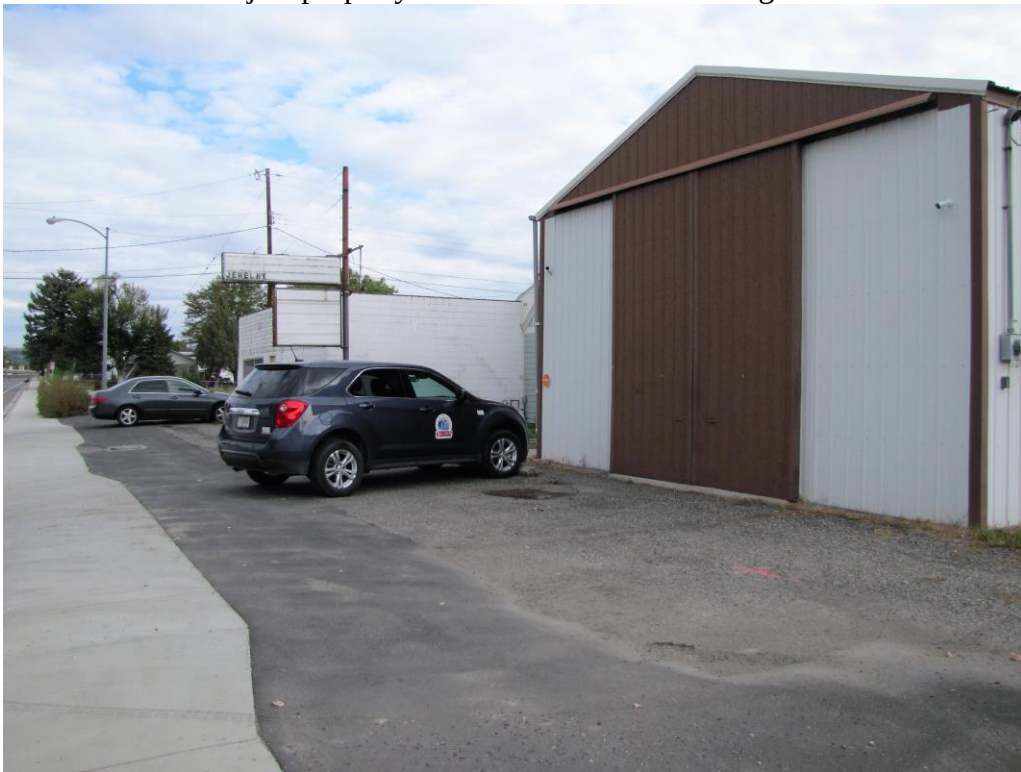
Looking north across existing buildings
