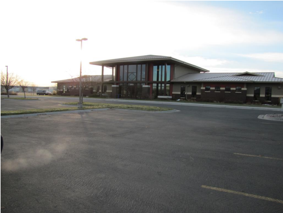
From North Property line looking at existing structure and parking area.
