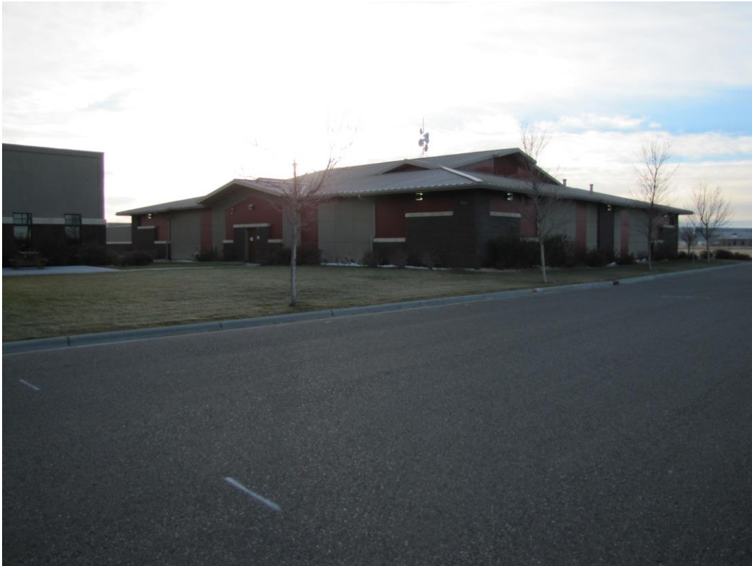
Looking from the north of the proposed lot line at the existing building to the south.
