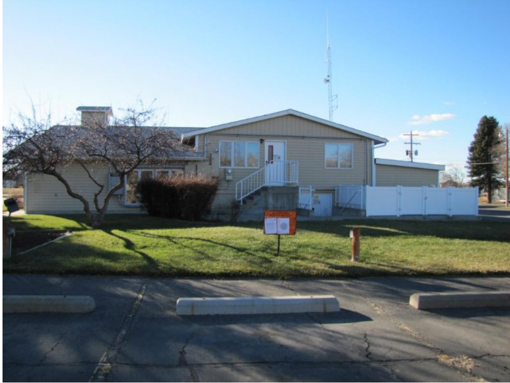
Subject property from McIntosh Drive
