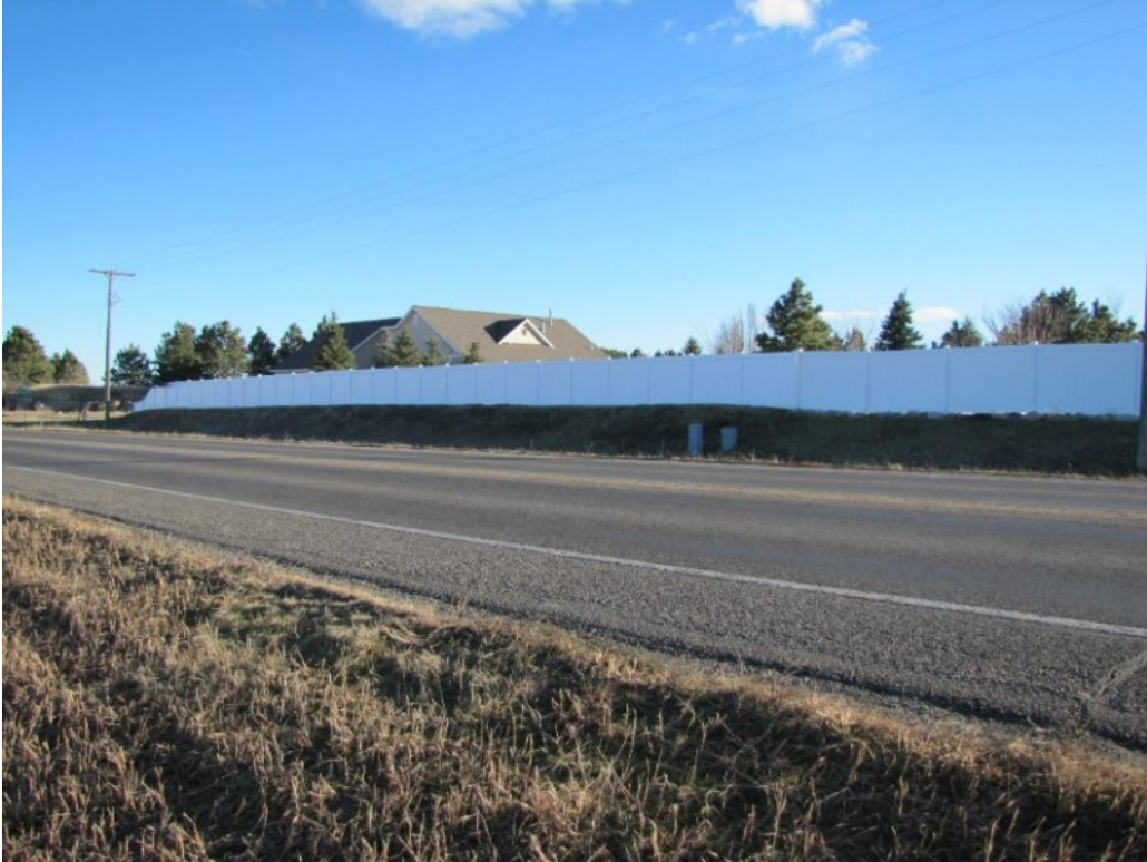
View south and east across Highway 3
