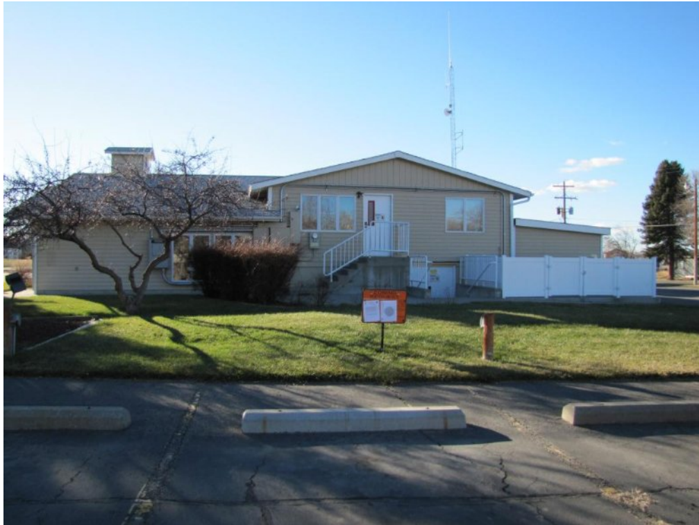
Subject property from McIntosh Drive
