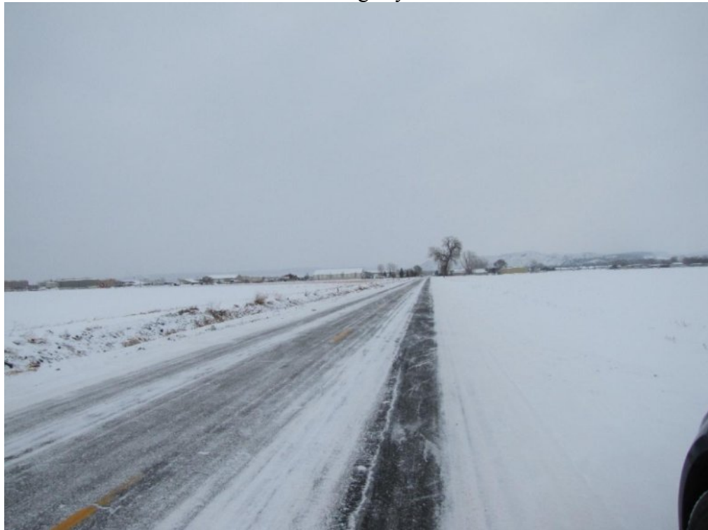
View east along Elysian Road
