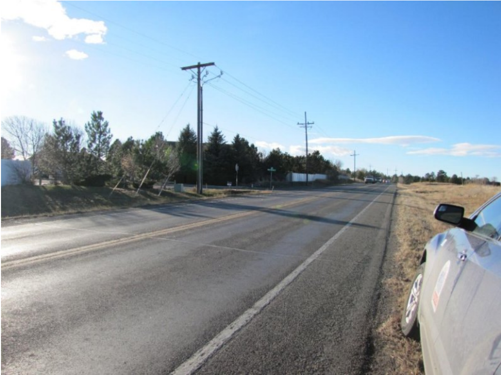
View west across Highway 3
