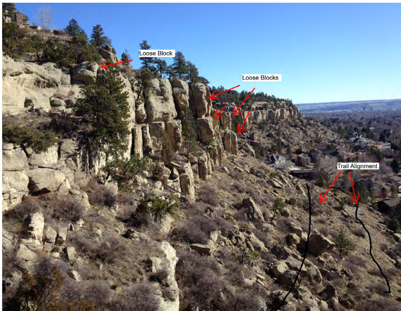
Looking east along cliff face above Sta. 20+00 to 24+00
