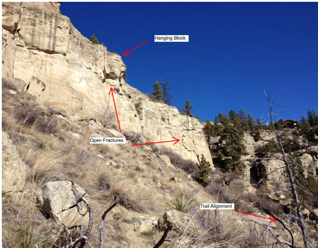
Looking north along cliff face above Sta. 25+00
